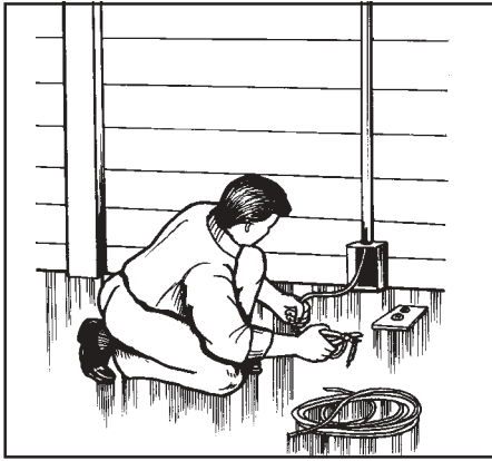
e. cutting cables without wearing rubber gloves
