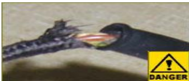
Electrical equipment with damage cord
